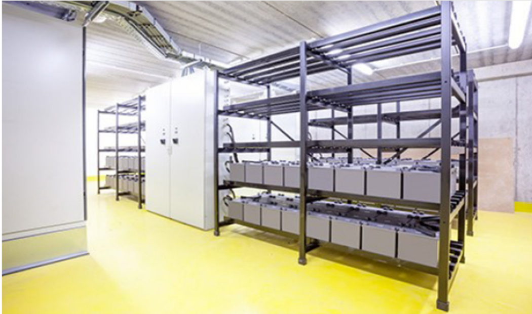
A room is being converted into a battery room and therefore requires an electrostatic dissipative (ESD) floor. With StoPox WL 213, this is no problem. Photo: denboma/Adobe Stock
