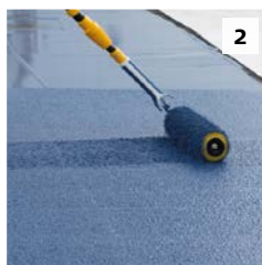
2 Roll StoPox KU 614 thix evenly in a criss-cross pattern. Tool: texturing roller medium-fine
