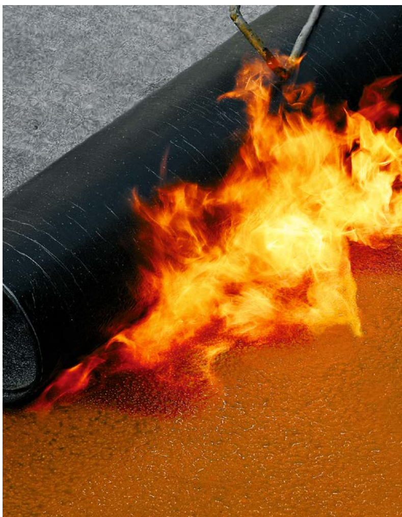
Bridge sealing with StoPox BV 100 and bitumen sheet
