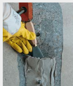
Removing the sealing
