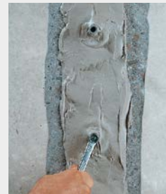
Screwing in the cone nipple
